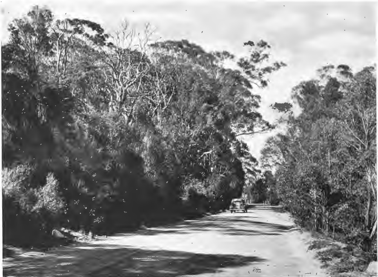
A section of the completed road at top of Mt. Tomah.
