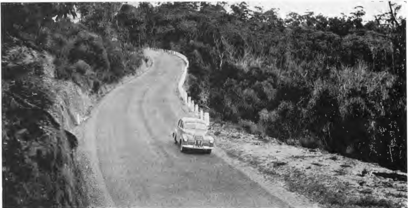
Completed section of road on the Kurrajong side of Bell.
