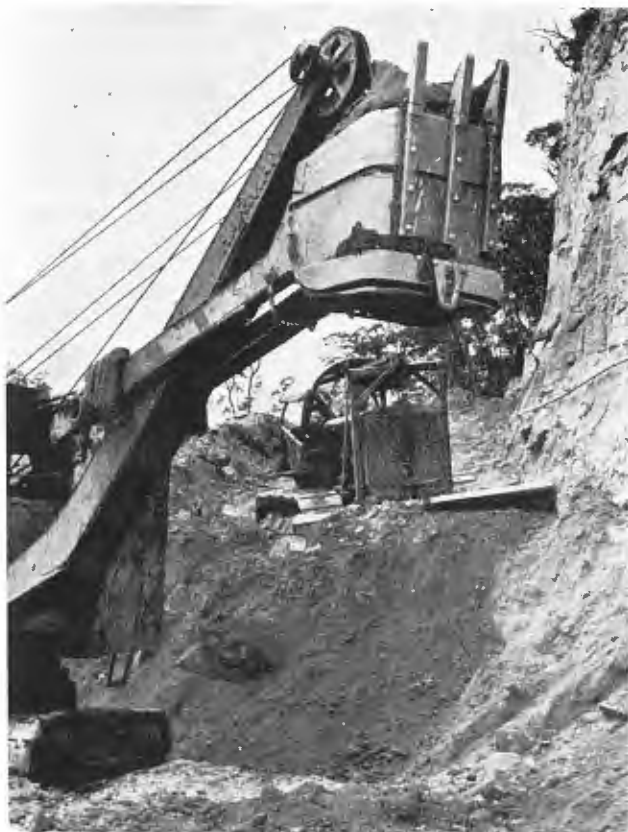
Shovel and Bulldozer at work.
