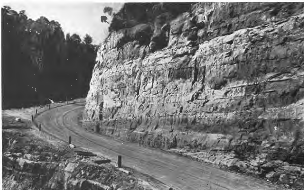
Completed work on cutting. (See photo. page 21.)
