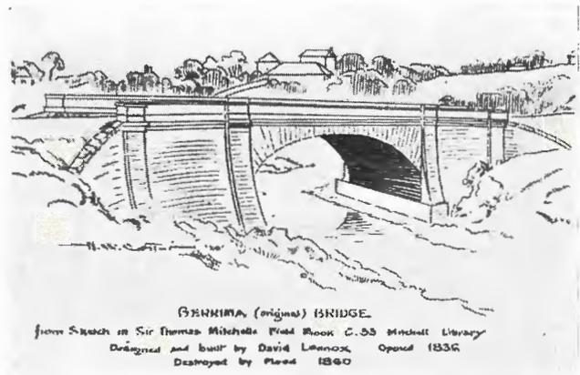
On the 23rd January, 1834, Lennox reported having laid out the site of a bridge on the main southern road at the crossing of Midway Rivulet, 3 miles south of Berrima. For this crossing a wooden bridge was designed supported by three masonry piers 20 feet apart. In 1835 the Surveyor-General reported that the bridge had been completed.
